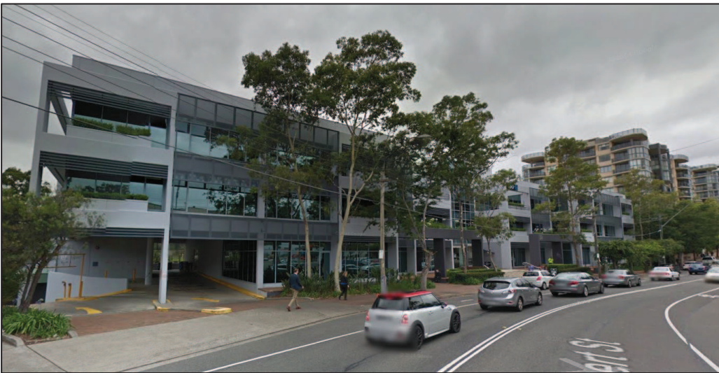
PICTURE 2 – AS VIEWED IN THE CONTEXT OF RESIDENTIAL TO THE SOUTH
